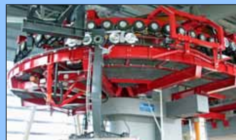
This massive wheel at the Whistler Terminal drives the gondola haul rope and the 28 gondolas attached to it.
