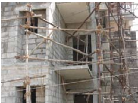
The view of the construction outside my back window.
